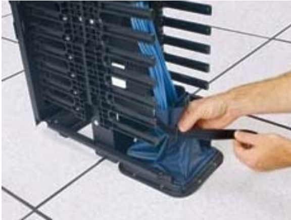
Figure 64: Gasket Seals Off Access Floor Tile Cutout In Vertical Cable Manager
